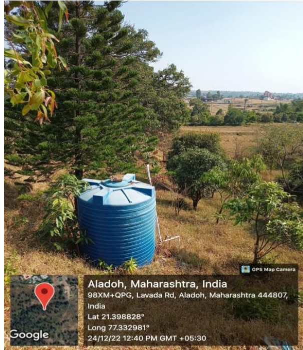
Constructed Water Tank For Garden at Aladoh campus
