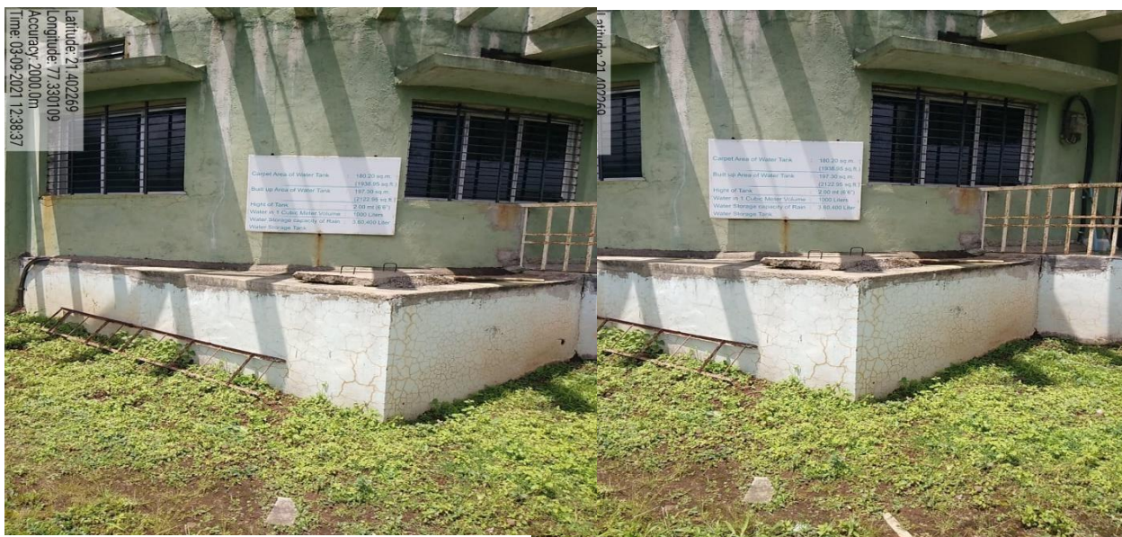
Water conservation facility available at college campus –Girls Hostel Building
