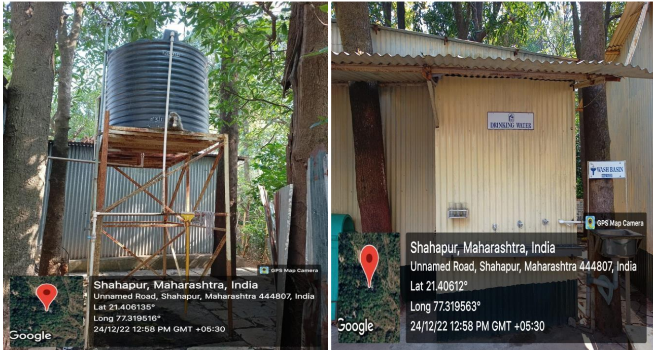
Water Tank for Drinking water at College Campus
