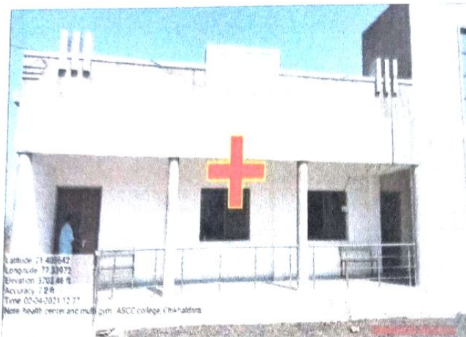
Health Center and changing room, Aladoh, Chikhaldara
