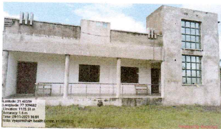
Multi Gym(indoor), Aladoh, Proposed Site, Chikhaldara
